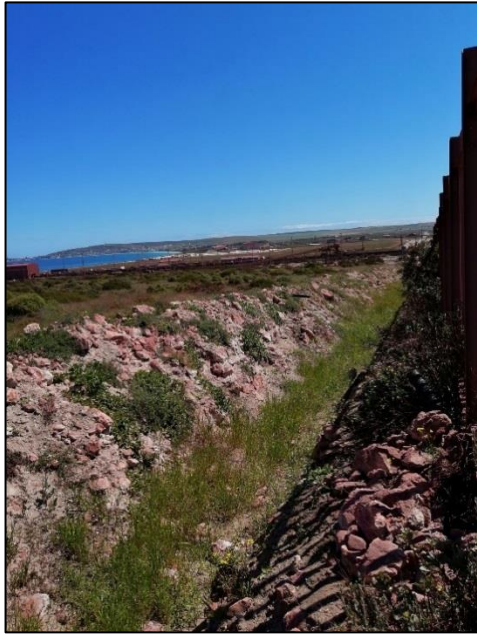
Figure 4: Excavated conditions of a portion of the inbound pipeline route
