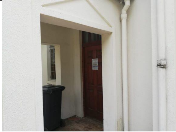
Figure 4 ST John's Anglican Church (Kerk Street Kylemore)
