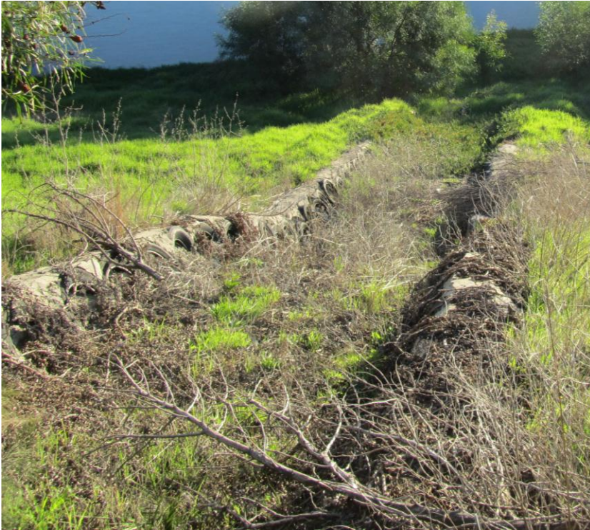
Figure 16. View of one of the drains into wetland area
