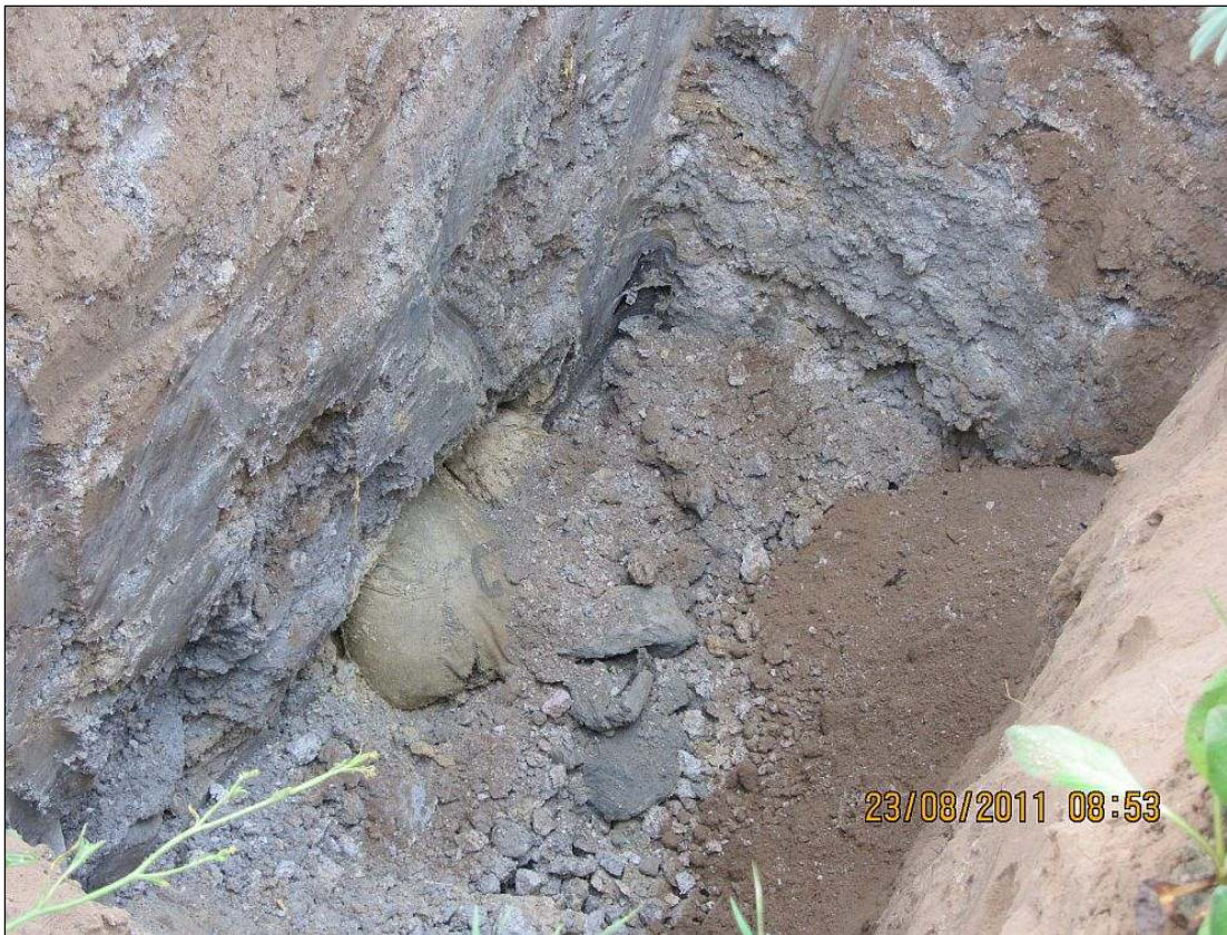
View of ASBESTOS SLUDGE in IP203. Note bags filled with ASBESTOS SLUDGE (slurry) at base of inspection pit.
