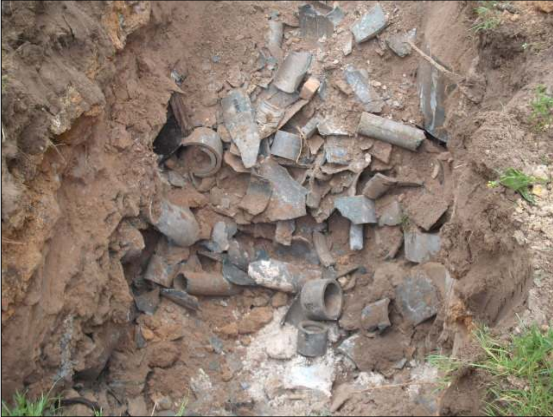
View of loosely packed asbestos pipes and other asbestos waste in IP228.
