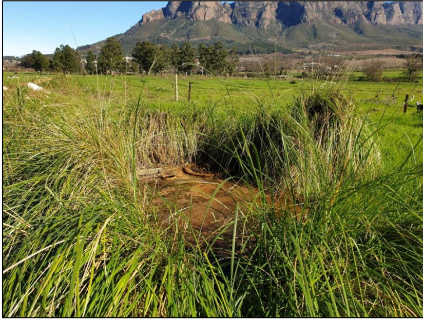
Figure 3.2 Air valve chamber in a pond that has developed around a leaking water mains pipe, adjacent to the New Retreat site. The leak feeds the seep wetland next to the site, artificially enlarging the wetland area.
