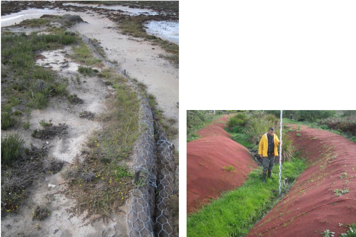
Figure 8.6 (Left) Ecologs used to stabilise the banks of a stream; (Below) Geotextile stabilisation of a slope.
