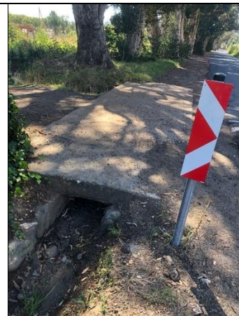
Figure 37 Closer view of culverts under the crossing to the pump station (2)
