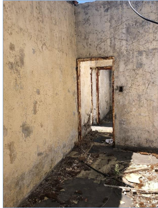
Figure 13 Inside one of the derelict cottages, note no roof and no internal facilities/furnishings (2)
