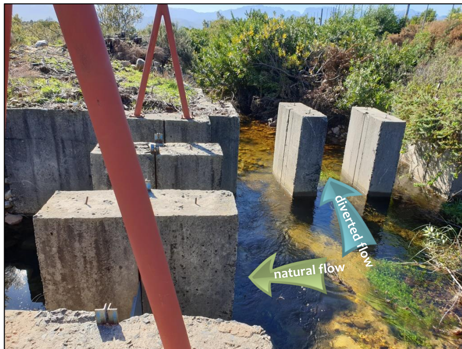
Figure 2.2 Diversion of surface flow from Stream 10 into the diversion channel flowing towards Normandie Dam. The sluice gates on the left were all closed at the time of the field visit in July 2020.
