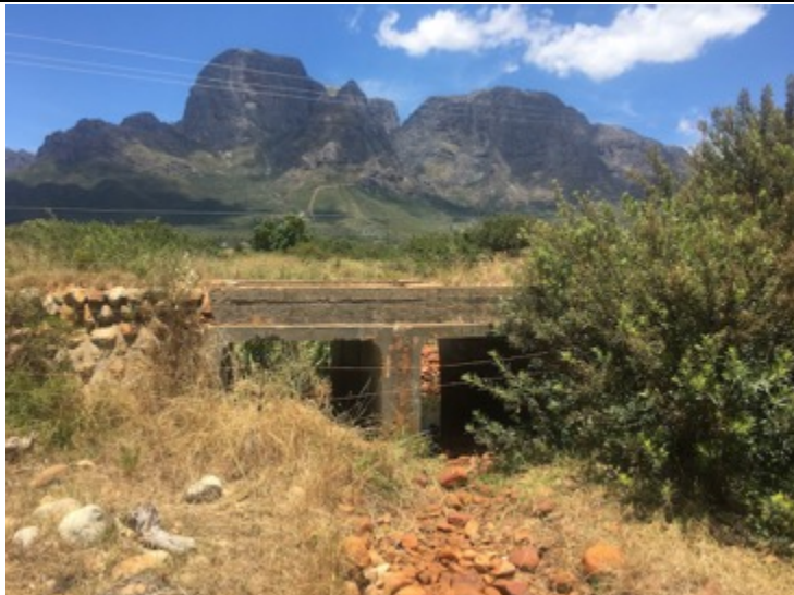
Photo 7: The existing double box culvert road crossing.
