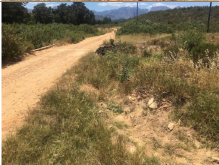
Photo 8: Another view of the existing road crossing. When the culvert surcharges, excess flows are likely to pass overland on either side.
