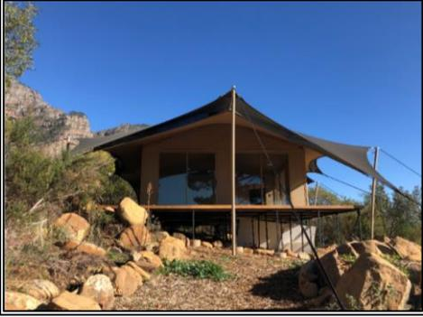
*Figure 19 Typical accommodation tent, note raised on steel frame supported by individual poles, composite wood-walling and stretch canvas roof*
