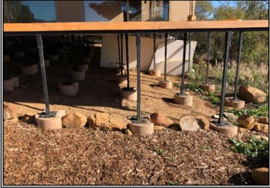
*Figure 20 Closer view of platform supporting accommodation tent*
