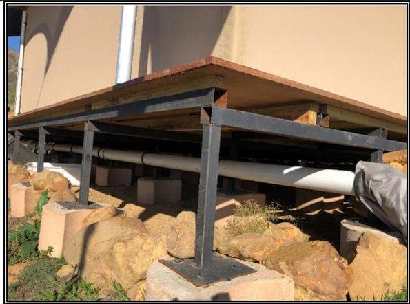
*Figure 4 Steel frame and supporting poles underneath office tent*
