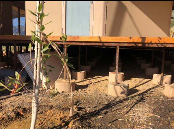
Figure 9 Supporting frame and poles underneath mess tent
