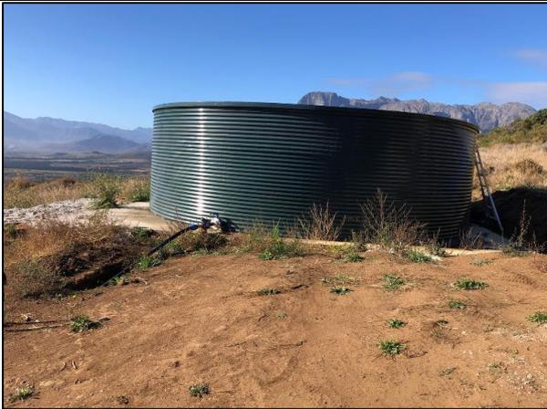
*Figure 35 Reservoir on concrete slab*
