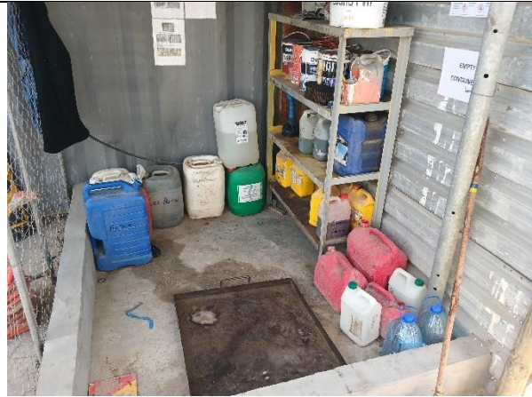
Photograph 32: Hazardous substances are stored in a bunded area.
