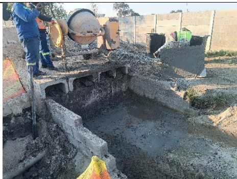
Photograph 39: concrete mixing area with sump to capture all run-off and cement.
