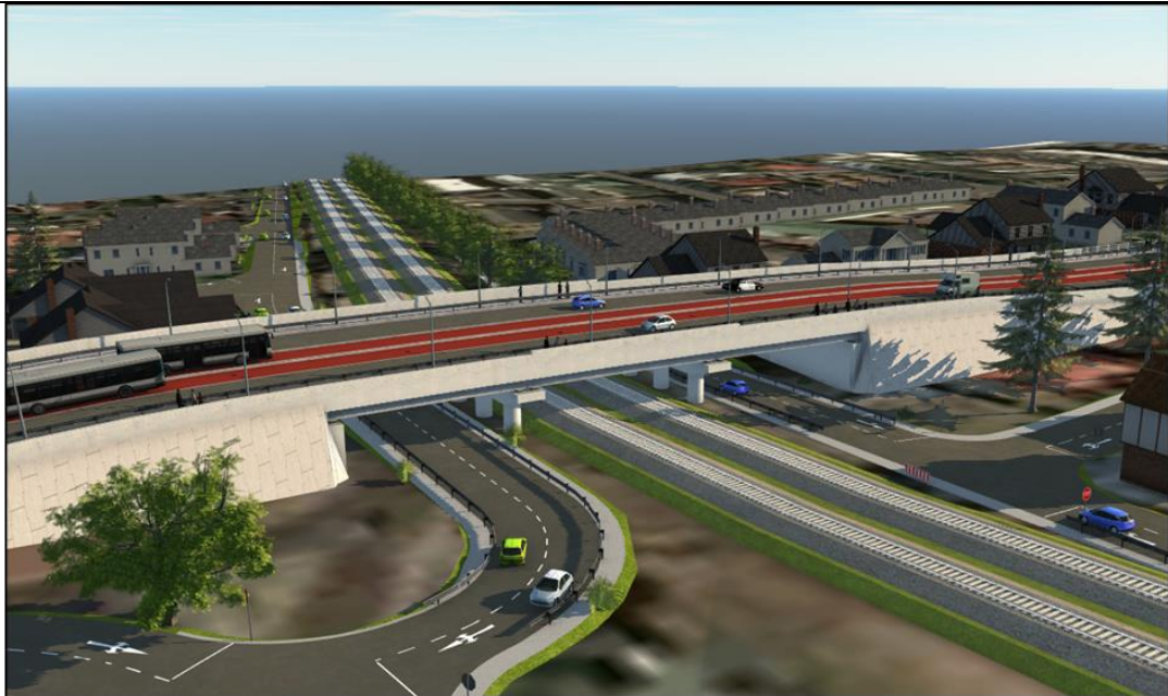
Figure 5: Conceptual view of three-span bridge (road-over-rail) (source : HHO Conceptual Design Review Report, August 2023)
