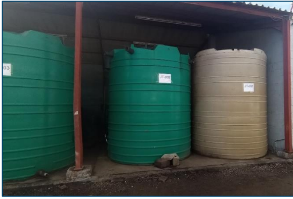
Figure 3: Impermeable tanks stored on site that house wastewater for storage prior to transport offsite
