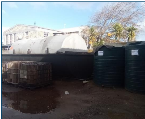
Figure 7: Used oil receiving storage tank located within the yard. The storage tank is bunded.
