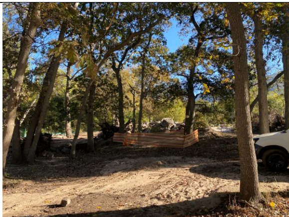
PHOTO 19: Tree protection fencing erf 212
