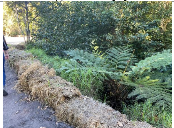
PHOTO 6: Hay bales for sediment trapping along the water course
