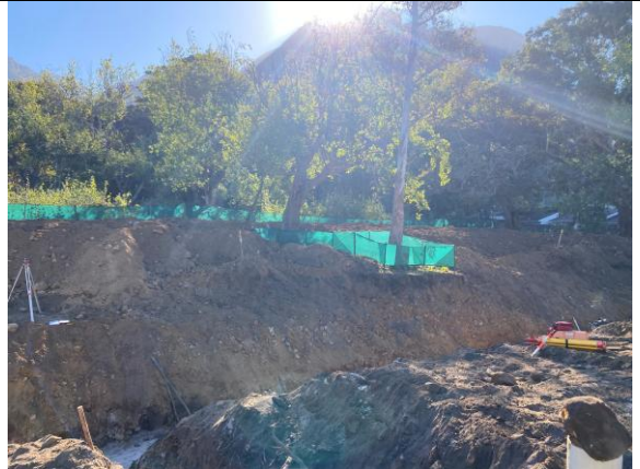
PHOTO 18: Tree protection fencing erf 242
