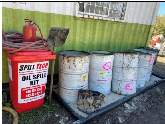
PHOTO 24: Good use of drip tray and spill kit on site
