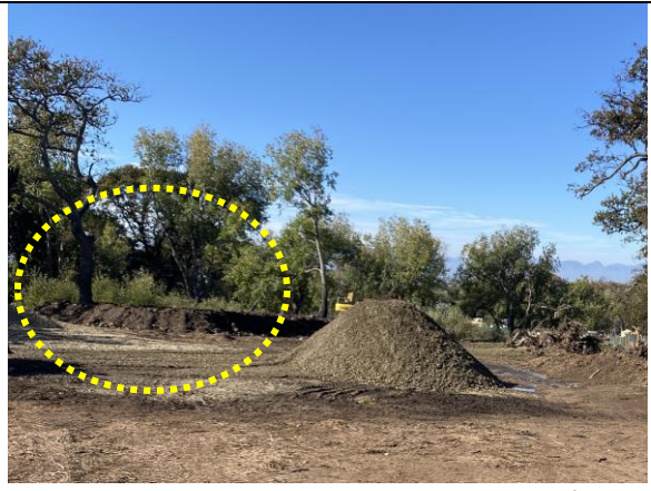
PHOTO 16: Soil stockpiling around tree base erf 242
