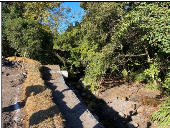
PHOTO 8: New gabions and hay bale sediment trapping on the edge of the water course
