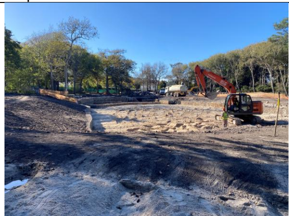
PHOTO 14: Stormwater ponds being built
