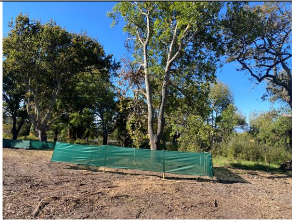
PHOTO 15: Tree protection fencing erf 242
