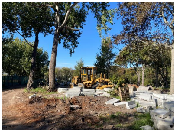
PHOTO 21: Kerb stockpiling around tree base erf 212
