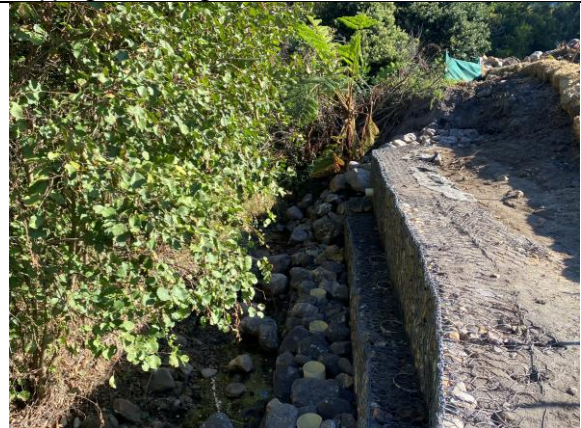
PHOTO 10: New gabions and hay bale sediment trapping on the edge of the water course
