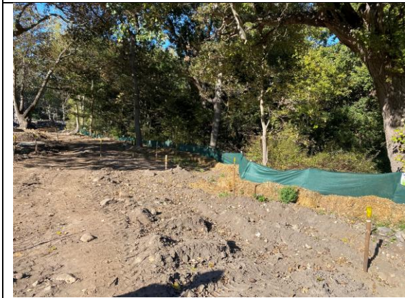
PHOTO 5: No-go area demarcation of the POS and hay bale sediment trapping is evident
