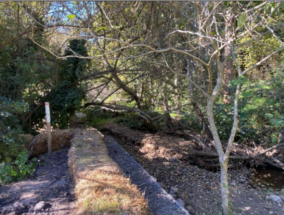
PHOTO 9: New gabions and hay bale sediment trapping on the edge of the water course
