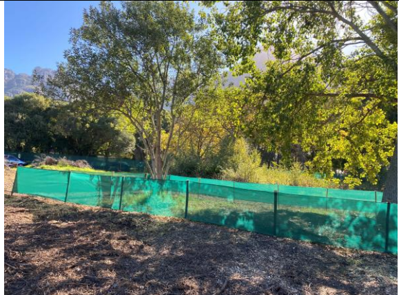
PHOTO 17: Tree protection fencing erf 242
