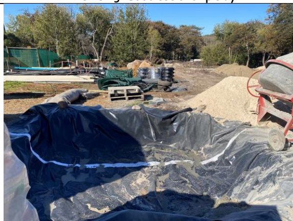
PHOTO 27: Good sump for concrete mixer effluent
