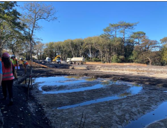
PHOTO 13: Stormwater ponds being built
