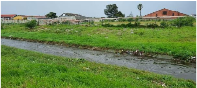
Figure 10: Watercourse adjacent to the site (captured on 27/08/2024)
