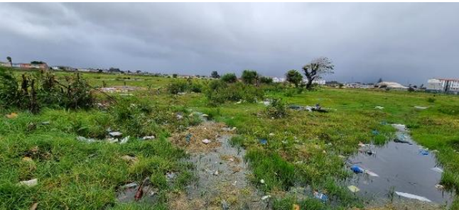
Figure 7: Ground conditions of the site (captured on 27/08/2024)
