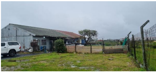
Figure 1: Existing structures on site (captured on 27/08/2024)
