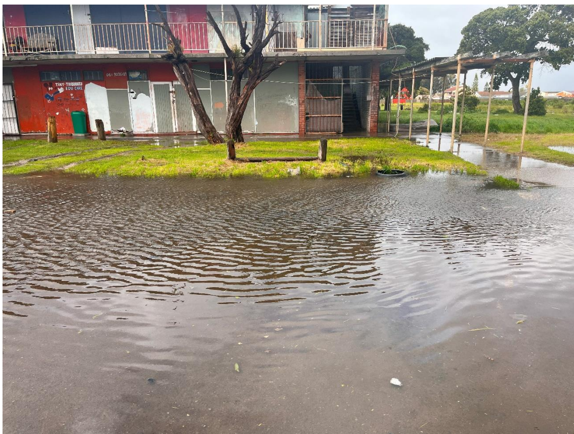
Photo 6: Flooding noted on site on existing paved areas
