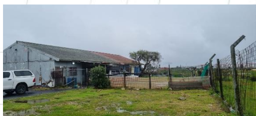
Figure 16: Old school building located within the proposed development site (captured 27/28/2024)
