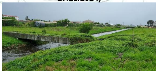
Figure 18: Big Lotus Canal located approximately 65m west of the proposed site (captured 27/28/2024)
