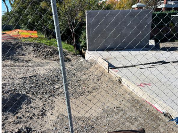
PHOTO 11: Culvert work site is clean and controlled. No stockpiling next to the culvert.
