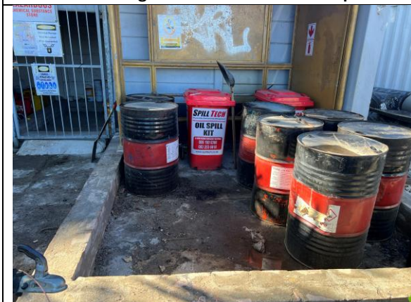
PHOTO 19: HCS storage and spill kit at the main site camp
