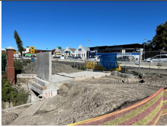
PHOTO 9: Completed culvert extension looking towards Imam Haron Road
