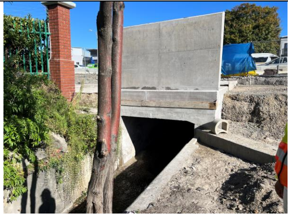
PHOTO 10: Culvert clean and clear
