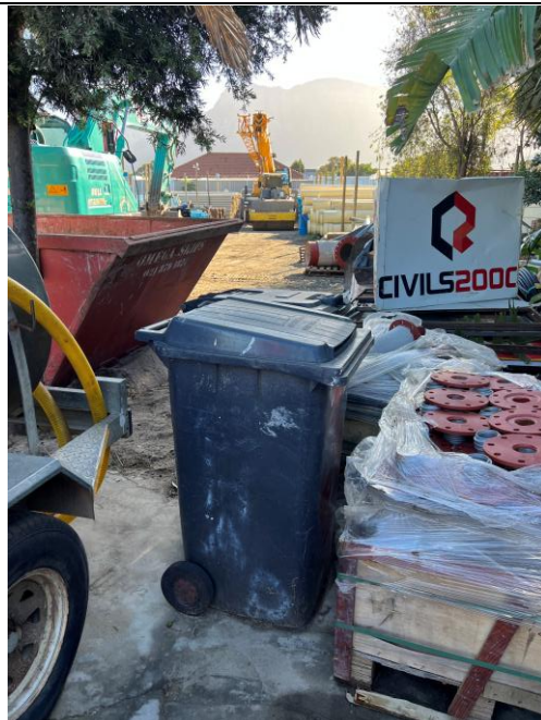
PHOTO 18: Skip and bin at the main site camp
