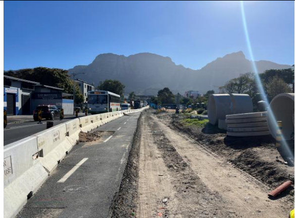
PHOTO 12: Controlled access/traffic management to work site and satellite laydown/facilities area.
