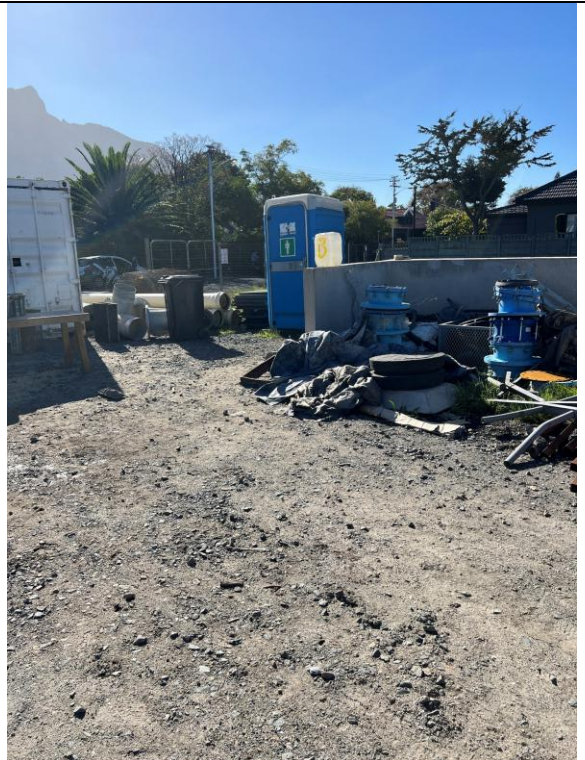
PHOTO 14: Satellite laydown/facilities area near the culvert work site. General waste bins, drinking/wash water and toilet facilities are provided.
